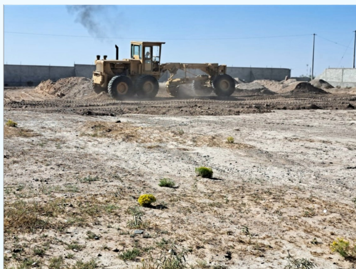
Leveling the ground for the school, Oct. 2023
